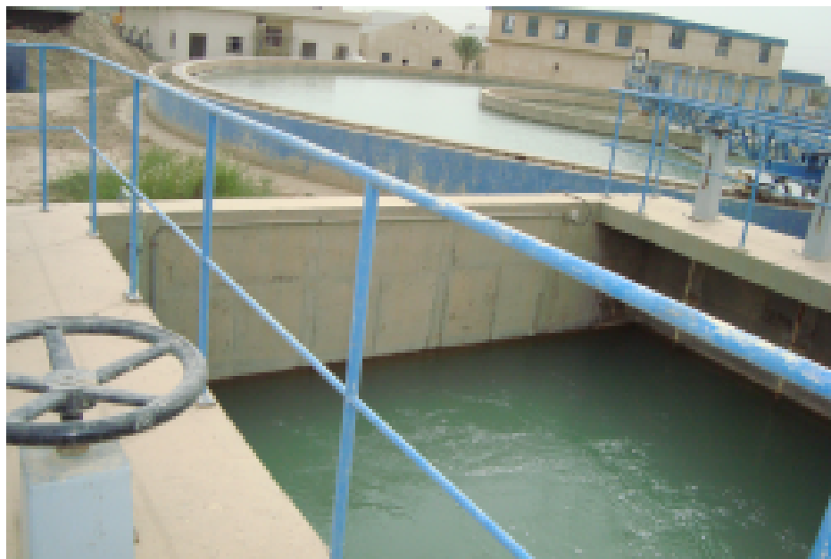
Figure 2. Coagulation and ClariFlocculator Tanks in DWTP
