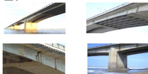
Figure 16. The view of bridge [42]
