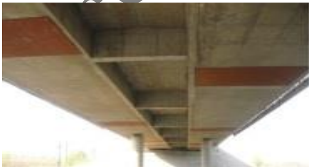
Figure 18. bridge structure after strengthening [43]
