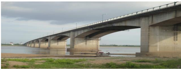
Figure 6. Actual structure of Jiamusi bridge [25]
