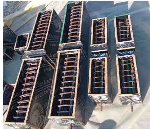
Figure 5. The wooden molds with the steel reinforcements.
